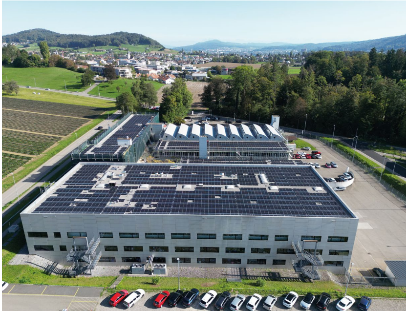
Huba-PV-Anlage-AEW_V01.jpg: A high-tech PV system is being built on the roofs of Huba Control AG in Würenlos on an area of approx. 3456 square metres.
